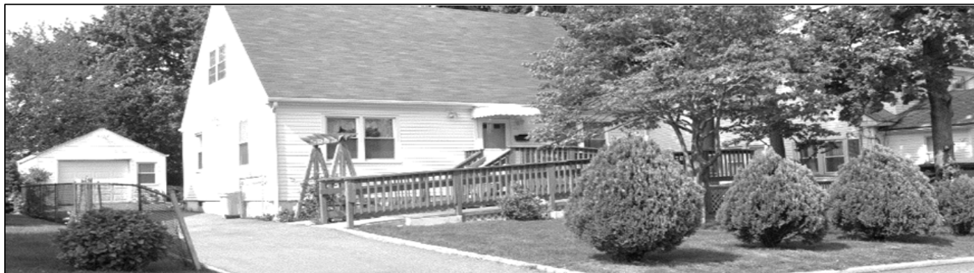
Pictured above: A white house with a driveway. A wheelchair-accessible ramp leads from the driveway to the front door.
